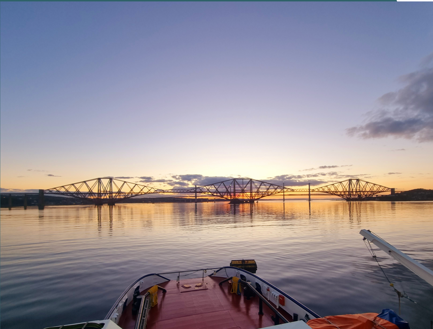
Forth Rail Bridge taken from Hound Point by Mark Costello
